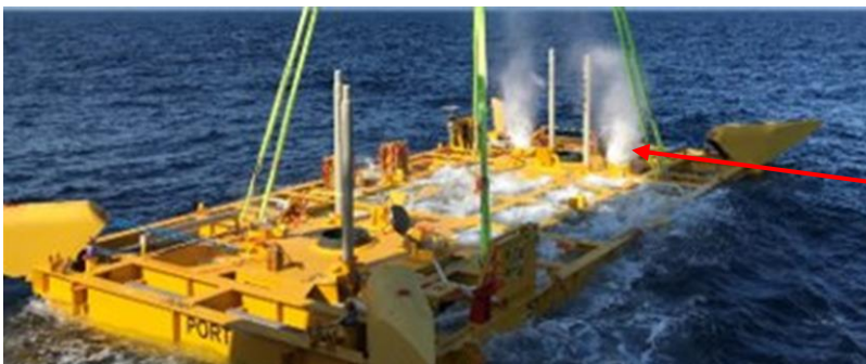
Template during installation with SubseaDesign delivered suction hatches
